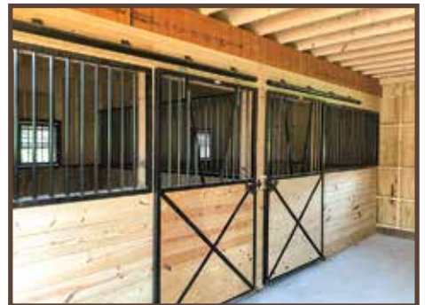
On-Site Build Horse Barn
