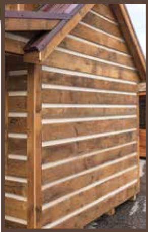
Old Reclaimed Siding with Chinking
