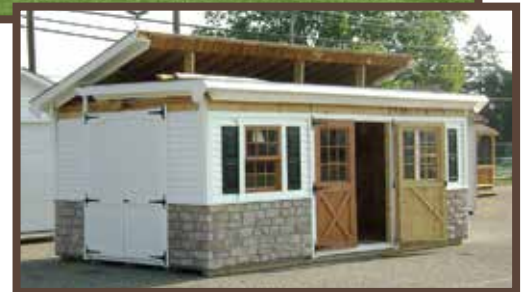
Hinged Gables and Hinged Roof Ready for Shipping
