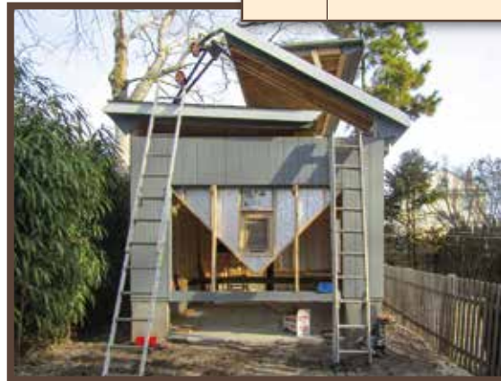
Jacking up Roof
