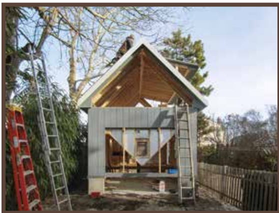
Hinge Roof Under Construction
