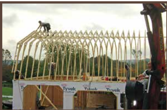
Build On Site
